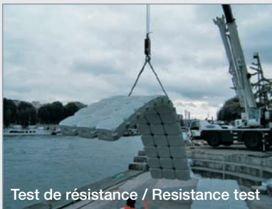
Barrage anti-pollution Anti-pollution barrier - Pillat, France
